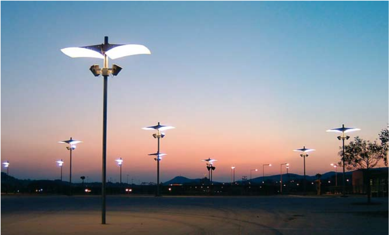
Fig. 1. Control gear with 3DIM functions taps into significant energy-saving potentials in street lighting applications
