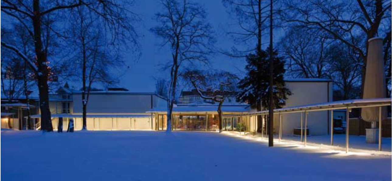
Fig. 1. The LED lighting in the park grounds of the Cardinal Wendel House conference centre in Munich creates a pleasant atmosphere
